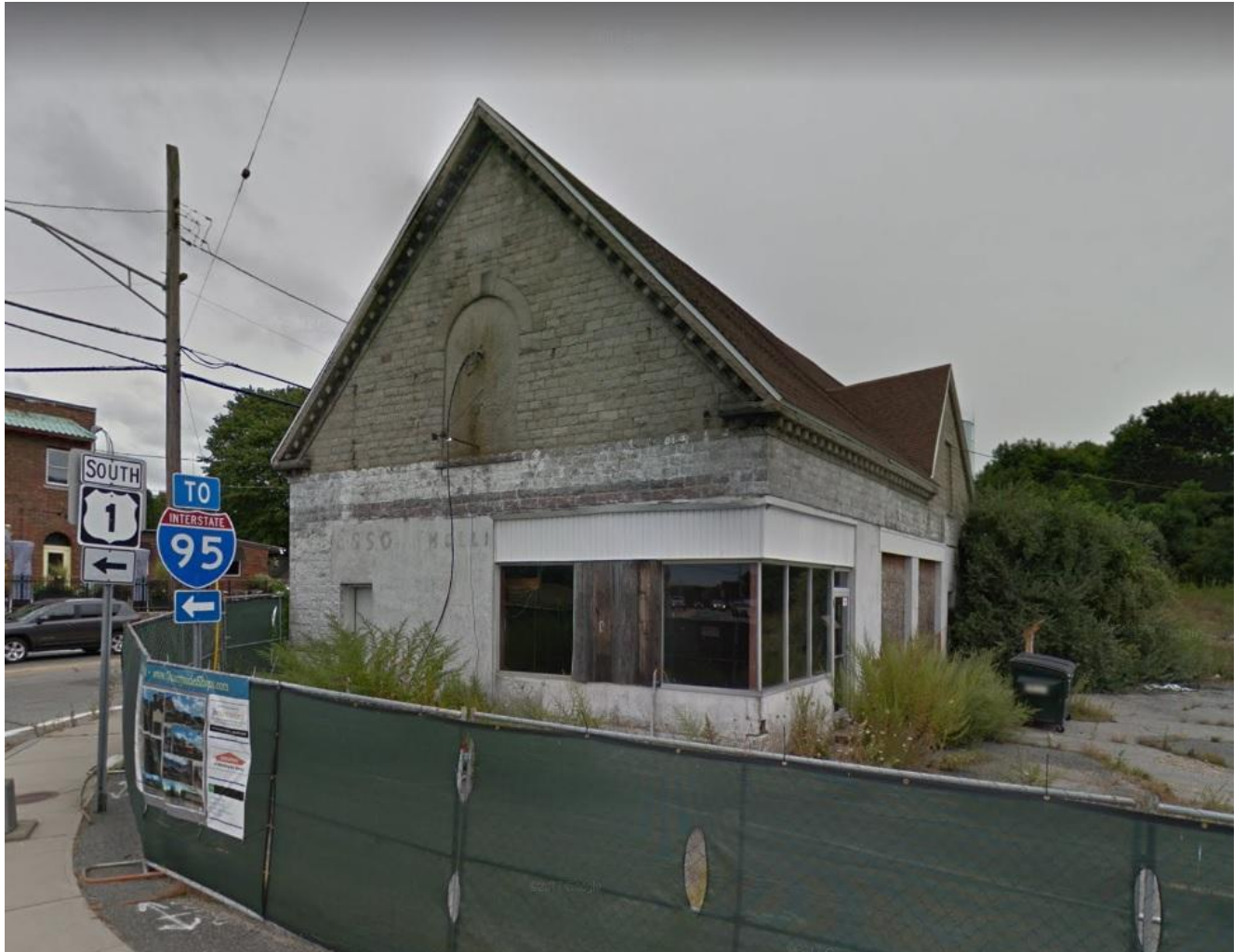
The site of Phil's dad's original dealership on Granite Street in Westerly. It appears that the building was undergoing some restoration at the time this Google image was taken.
